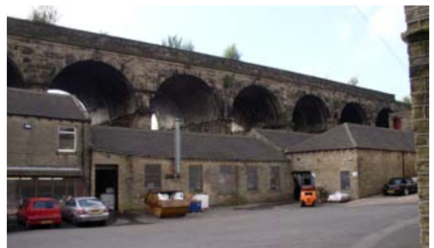
This is the Process Measurement and Analysis Ltd Factory
